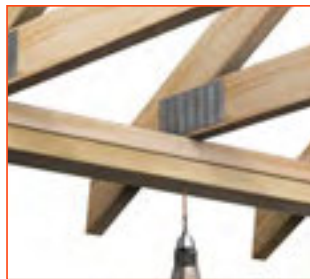
DOUBLE TOP PLATE TO TRUSS
