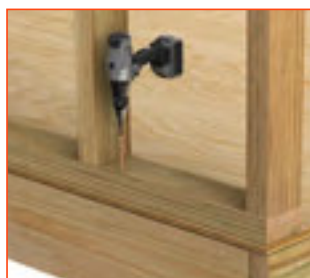
BOTTOM PLATE TO RIM BOARD
