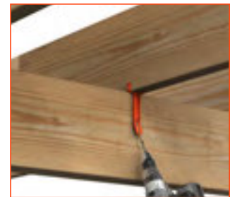
BEAM TO JOIST
