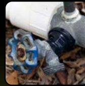
Repairs loose or leaky plumbing
