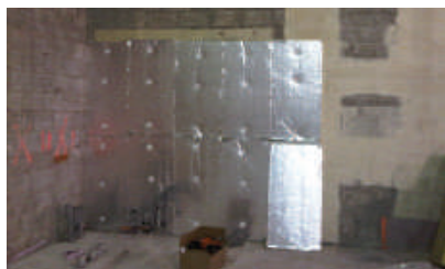
Interior walls on concrete block
