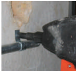
12HSMPO34 clip assembly used to secure conduit
