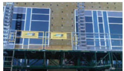
Behind cladding over steel stud walls
