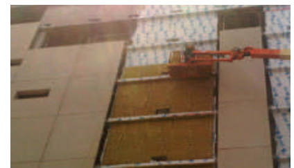
Behind cladding over concrete block walls
