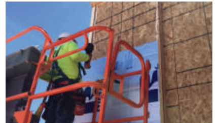
Behind cladding over wood stud walls
