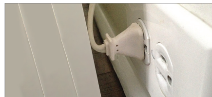
Within electrical cords accidentally damaged by furniture resting or pressing upon them
